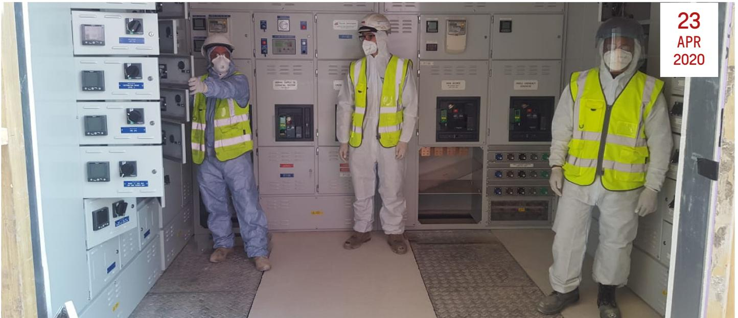
The switchboard had to be designed around a very tight new switchroom to provide supplies for all of the new services required for the GICU. It is also equipped with facilities to enable a portable mobile generator to be connected very quickly in an emergency. Facilities have also been incorporated to provide automatic changeover to an Emergency supply in the event of a main supply power failure.
